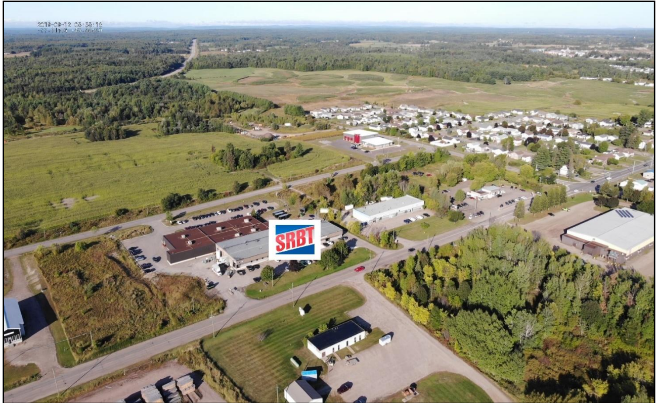
FIGURE 5: AERIAL PHOTOGRAPH LOOKING NORTHWEST OF SRBT FACILITY
