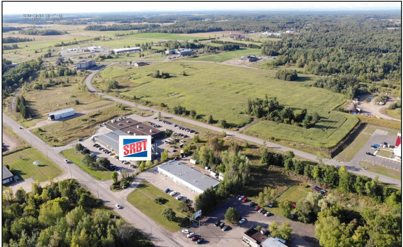
FIGURE 4: AERIAL PHOTOGRAPH LOOKING SOUTHWEST OF SRBT FACILITY
